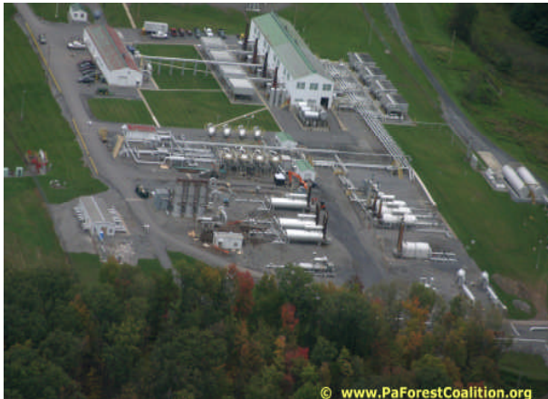
Compressor Station in the Susquehannock State Forest
